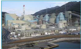
Maizuru Power Station (Coal fired power plant)
