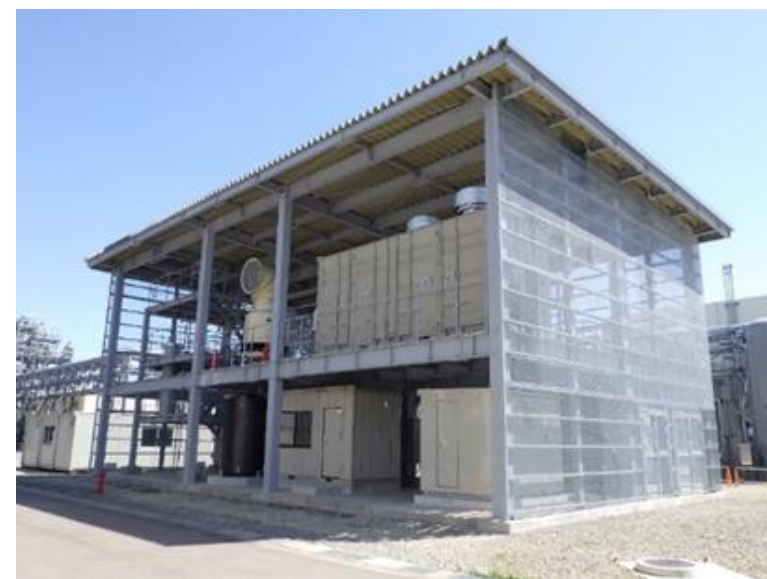
Methanation test facility (Pilot-scale: 8 Nm 3 -CH 4 /h, at Nagaoka, Niigata)
