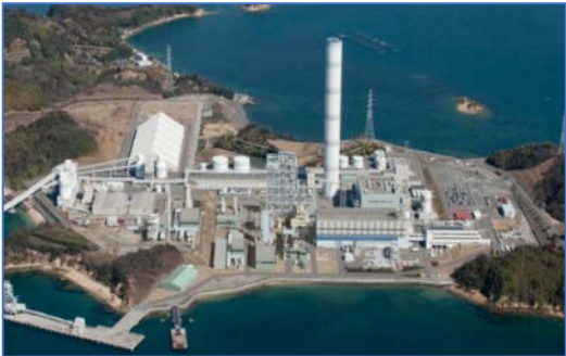
IGCC with CO2 capture and carbon recycling facility
